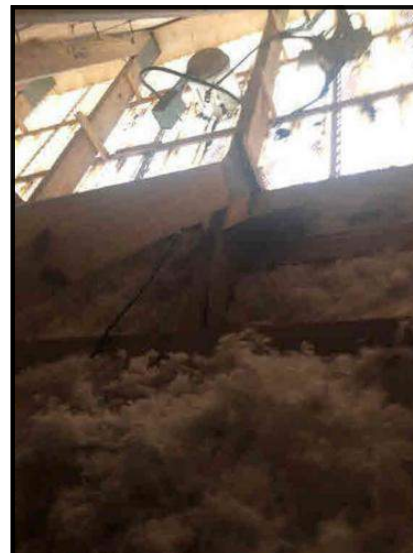
NOT ALL TRUSSES HAVE ATTACHMENTS
