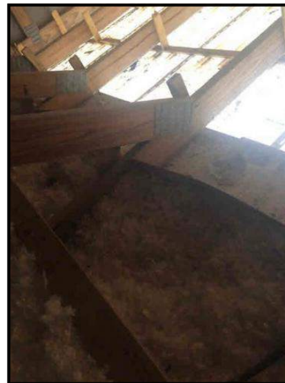
NOT ALL TRUSSES HAVE ATTACHMENTS
