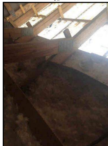
NOT ALL TRUSSES HAVE ATTACHMENTS
